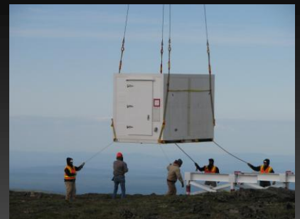
AK Supply Inc crew guiding the building to it's foundation
